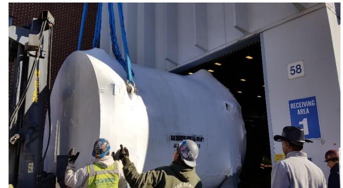
Moving the cryostat into the Test Lab with a door height of 13' 6"
