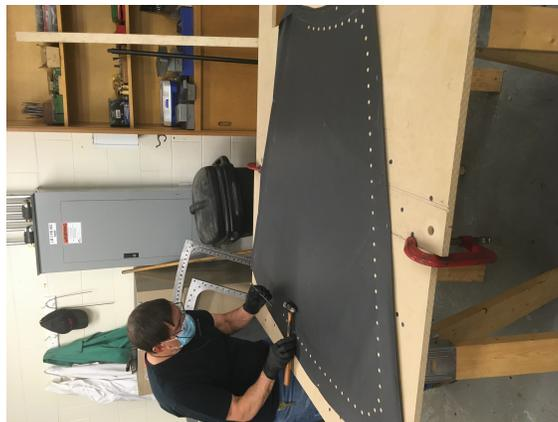
Figure 27: The Tedlar's bolt holes being punched.
